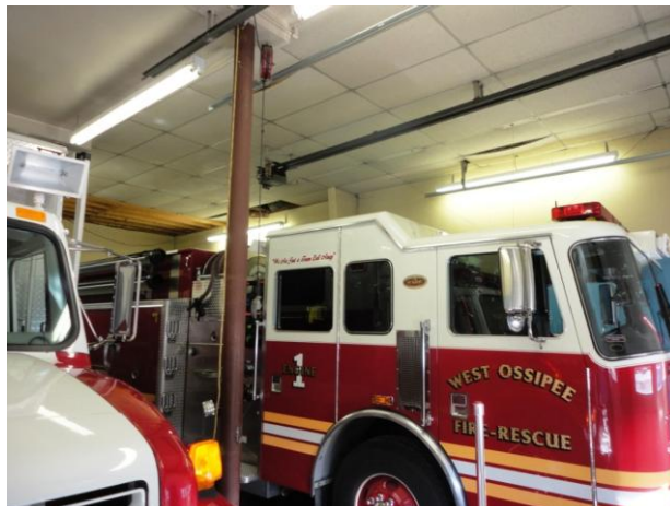
Figure 9. Apparatus Bay lighting
