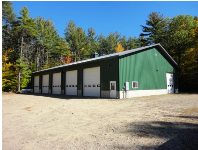
Figure 1. West Jewell Hill Fire Station
